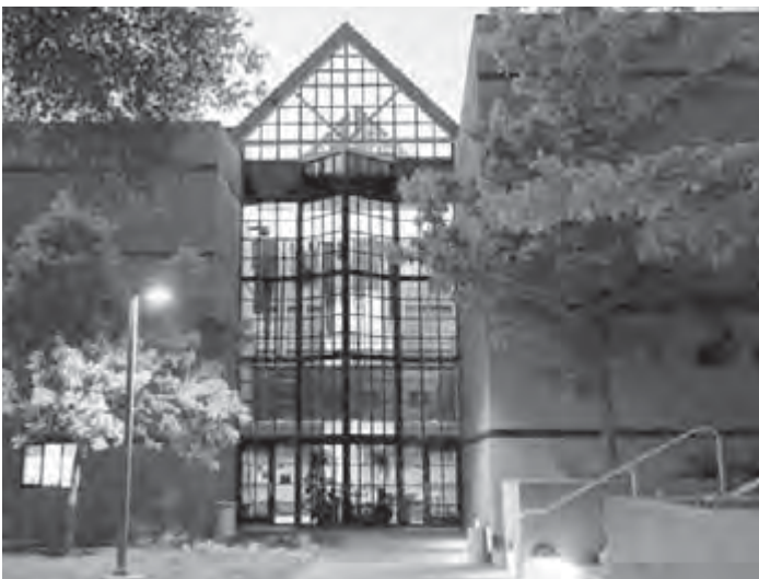
Building A at the El Dorado Center
