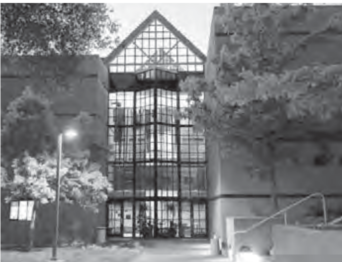
Building A at the El Dorado Center
